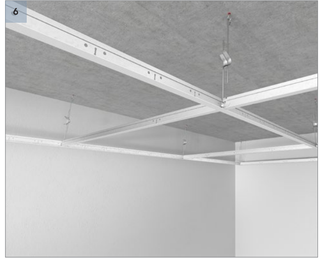
Install cross tee Click T24 1200 mm to main runners every 1200 mm.
